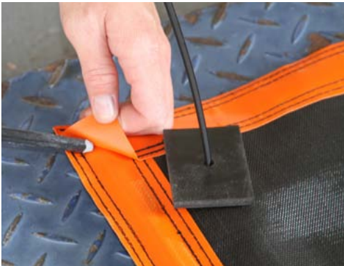
Step 3: Insert one of the included support rods in the opening threading it all the way into the sleeve.
